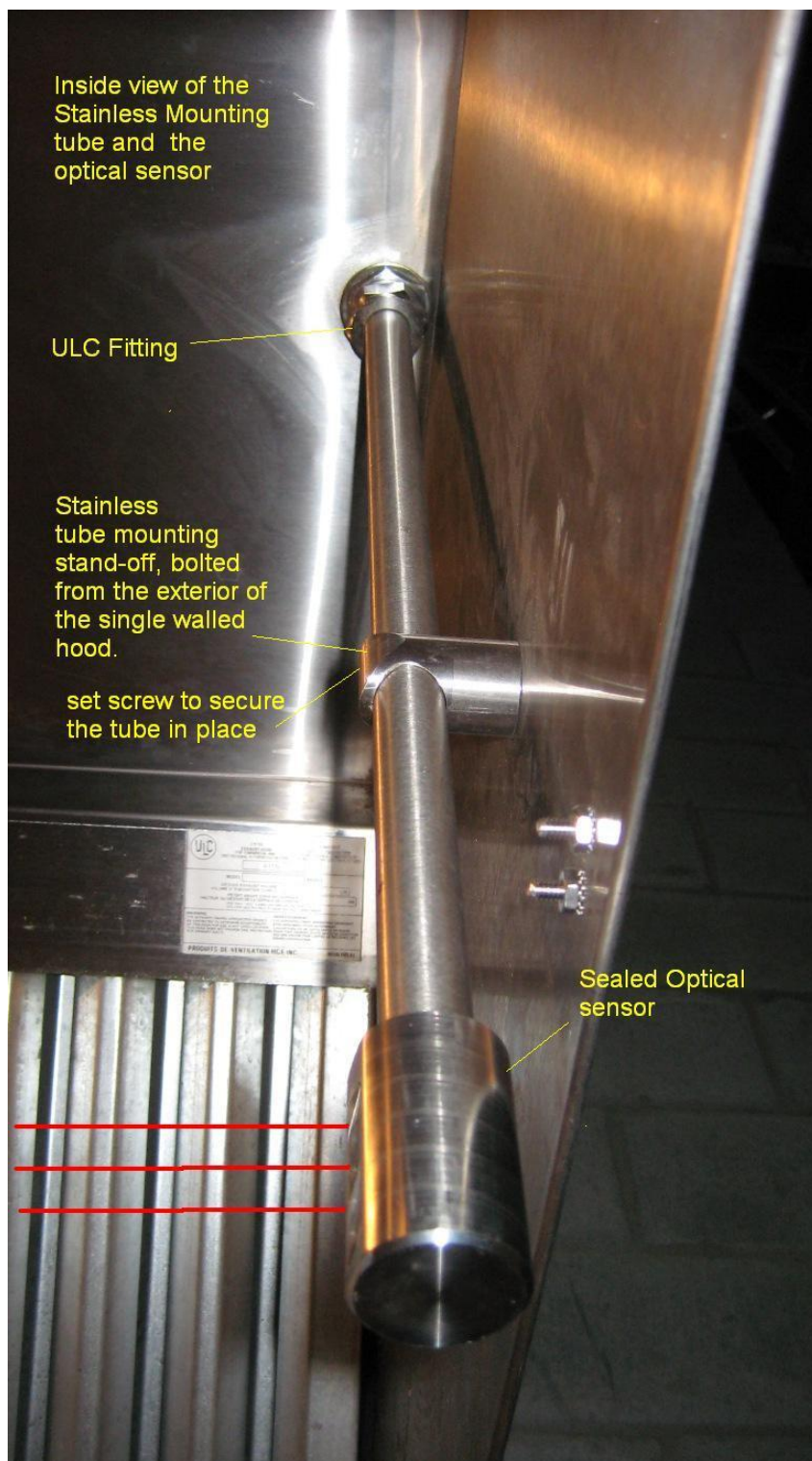
TYPICAL OPTICAL SENSOR INTERNAL MOUNT DETAIL
